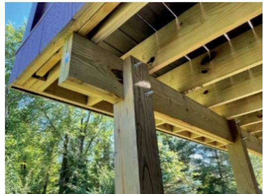
Notched 6x6 posts with double or triple 2x10 beams using a thru-lock system to tie the beam and posts together.
